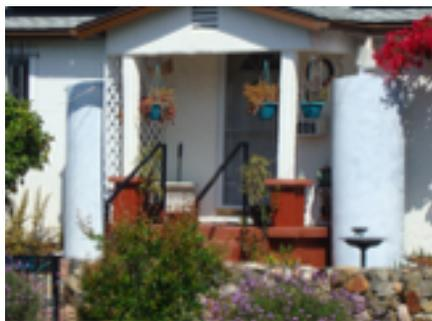
So the Dolphins installed two, 250-gallon water tanks on either side of their entry porch. Painted to blend right into the stucco exterior of the house, the tanks gather rainwater off the roof and provide all the irrigation water the Dolphins need for their lovely front yard and vegetable garden.
